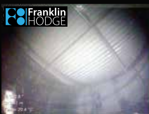
Underside of tank cover
