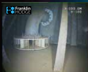
Anti vortex device & suction pipe
