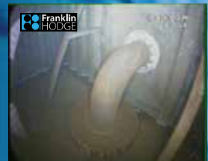
Tank floor area & fittings
