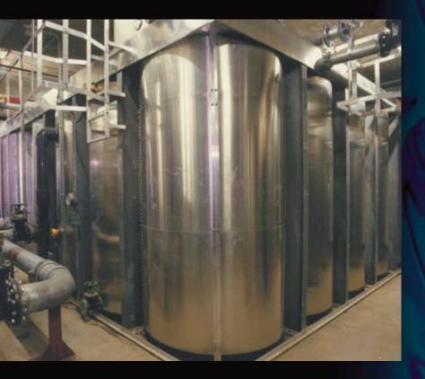
Versatility in design. A variety of shapes and sizes can be supplied. Existing obstructions such as building support columns can be encapsulated within the tank by 'sleeving' the membrane liner around them.
